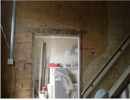
Figure 5: Stairway and previous entry to living area
