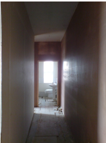
Figure 8: landing after walls were skimmed
